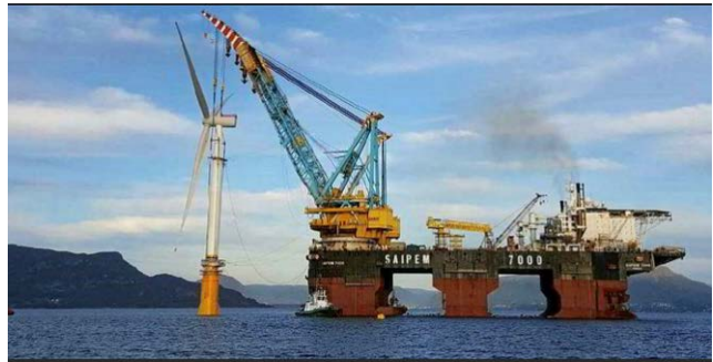
Figure 7 Lift of turbine onto Spar (courtesy Saipem)
