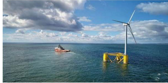
Figure 3 Semi submersible (courtesy Principle Power)
