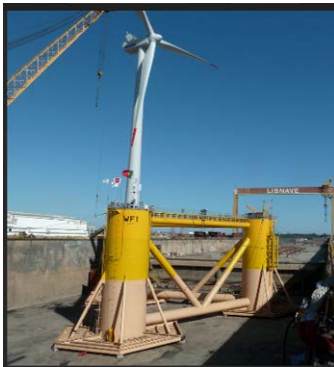
Figure 9 Semisub in drydock (courtesy Principle Power)
