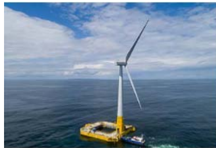
Figure 4 Concrete Ring Barge (courtesy Ideol)
